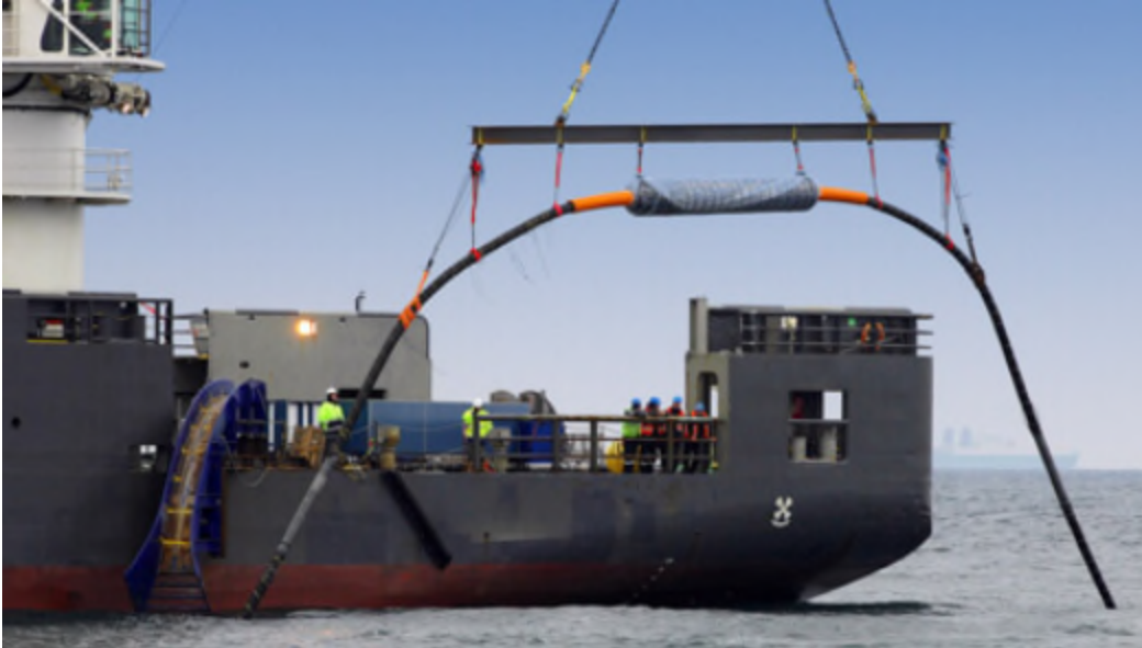
Figure 10.3-10: Vessel lowering an offshore cable joint using a bow.
