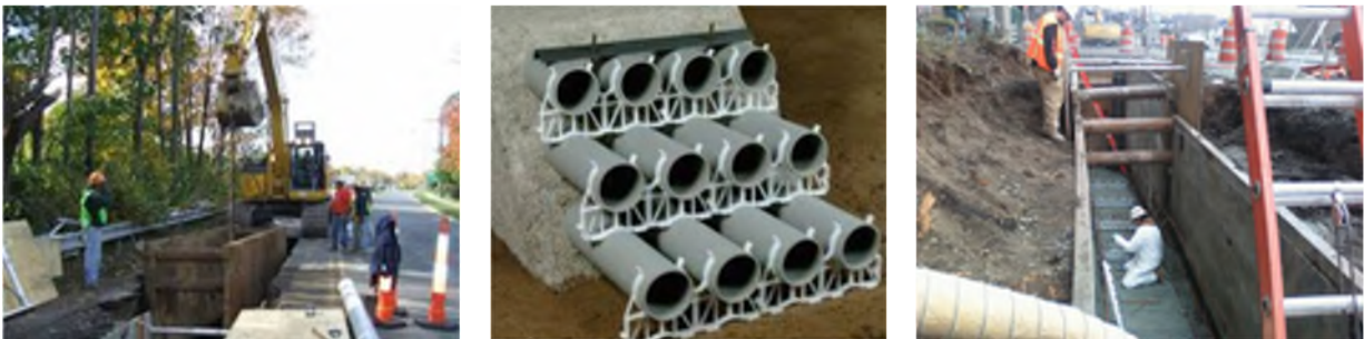
Figure 10.3-15: Onshore open trench and duct bank.
